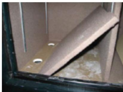
2. Drill a 1/4" hole in each of the 4 anchoring locations with a drill using a 1/4" wood drill bit approximately 2 1/2" to 3" deep.
